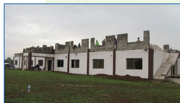
LICC second floor construction has begun
