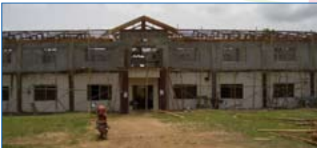
Schools Ready for its Roof
